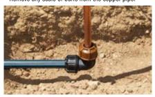
6. Remember to replace the stainless steel grip ring if re-using the copper connection.
