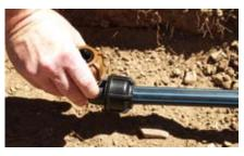
2. Tighten the nut by hand ensuring the nut flange is touching the fitting body, use a wrench if necessary.
