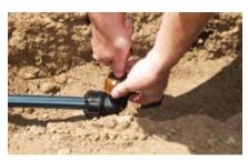
Tighten the nut by hand and finish using a wrench. Remember to check that the nut is tight against the body flange.
