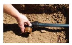
1. Cut PE or poly pipe square and insert until pipe stop is felt.
