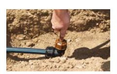
4. Insert the copper pipe and push into the rubber seal up to the mark indicated.
