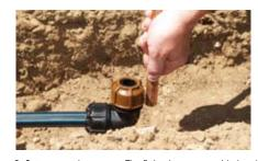
Cut copper pipe square. The fitting is pre-assembled and ready to use. Mark the depth of copper insertion using 'pipe stop' marking or body flange as visual indicator. Remove any scale or burrs from the copper pipe.
