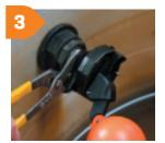
Valve body is suitable for final tightening with a wrench/multigrips to ensure perpendicular.
