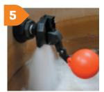
Ensure valve is perpendicular and turn on the water supply
