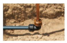
6. Remember to replace the stainless steel grip ring if using the copper connection again.
