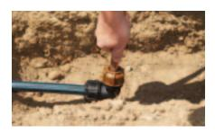
Insert the copper pipe and push past the rubber seal up to the mark indicated.
