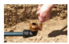
Cut copper pipe square. The fitting is pre-assembled and ready to use. Mark the depth of copper using pipe stop marking or body flange as a visual indicator.
