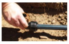
2. Tighten the nut by hand ensuring the nut flange is touching the fitting body, use a wrench as necessary.
