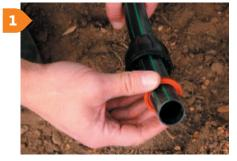
Cut the pipe square and place the nut and grip ring on to the pipe.
