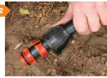
Tap the insert fully into the pipe.
