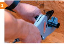
Cut the pipe square, there is no need to chamfer or lubricate the pipe.
