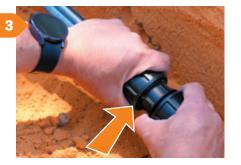
lighten the nut by hand to the point where the nut is touching the flange on the body of the fitting. Do not tighten beyond this point.
