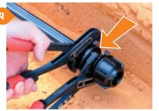
to 63mm may require the use of a wrench or multi-grips to tighten the nut so it is touching the flange.
