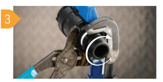
Using a pipe wrench or multigrips on the end caps only, further screw the ball valve until tight. Where necessary, ensure the thread is held stationary. Do not use pipe wrench or multigrips on the body of the valve.
