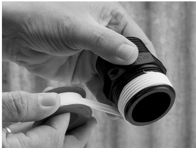
1. Apply PTFE tape or approved sealant to the male thread the blue handled ball valve is to be screwed in too. Sufficient tape needs to be applied to ensure a watertight seal
